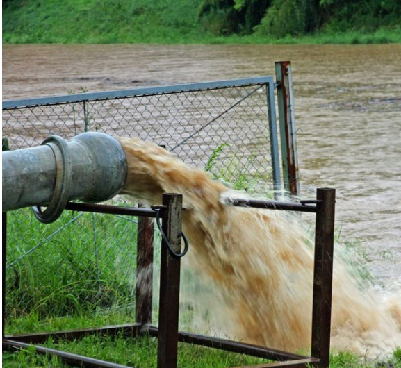
Site-specific waste volume quantification
